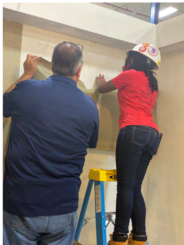
Mylenn is learning how to correctly install wallpaper.
